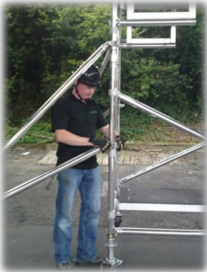
9. Secure stabilizers as soon as possible to increase tower stability.
