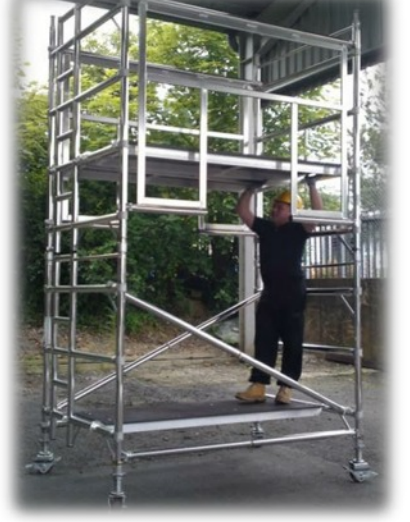
8. Position the trapdoor platform to the appropriate rung (Trapdoor facing the ladder section) 1 rung above the bottom section of the AGR frames.
