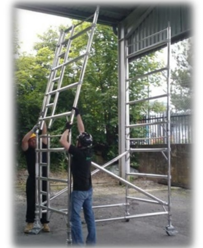
4. Add next level frames – according to your kit list.
