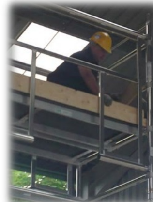
16. Fit toeboards in the correct position.
