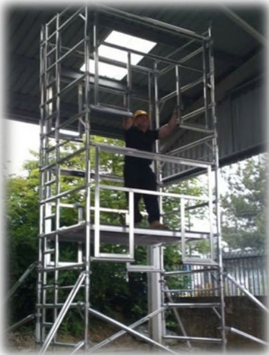
13. With the green label facing you, position the AGR frames to the vertical members, above the rungs in the required position as shown.
