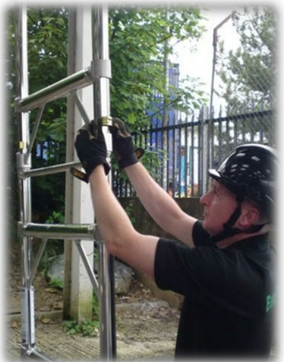
5. Engage Interlock Clips.
