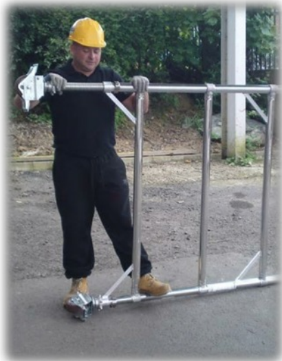
1. Insert 2 legs and castors into each frame.
