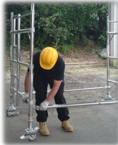
2. Klik in 2 horizontal braces to the vertical member of the frames, as low as possible, below the 1 st rung.
