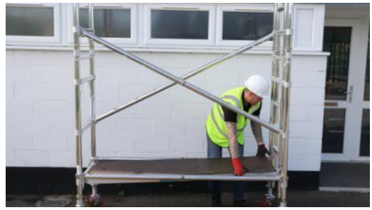
8. Fit 1 plain platform on the appropriate rung(see base builds). Level your tower by the adjustable legs using a spirit level as a guide. The scaffold must be verticle in both planes within an inclination of 1%
