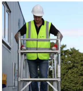
Unclip the 4 top hooks ensuring they do not re-engage. the trapdoor platform.
