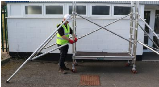
9. Fit 4 stabilisers at earliest opportunity keeping lower arms as horizontal as possible ideally 45 degrees.Stabilisers are fixed onto the frame uprights in each corner by the attached couplers.
