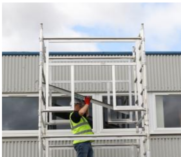
From the platform below, you can now remove both platforms above.
