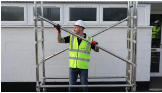
7. Fit 2 diagonal braces from the 2nd rung to the 4th rung in an alternate pattern.
