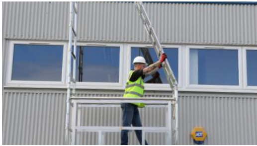
15. Continue erecting tower to final tower height repeating the AGR process as illustrated. Always ensure there is side protection to prevent falls. Platforms should be every 2m complete with handrails.
