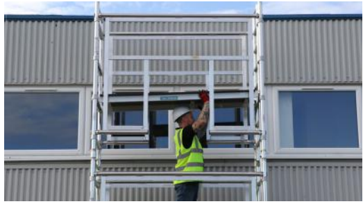
14. Fit 1 trap and 1 plain platform to the 3rd rung down. Making sure the trapdoor is with the ladder section.
