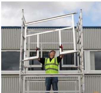
Unclip the bottom hooks of your AGR frames and remove. Be careful not to re-engage your top hooks.
