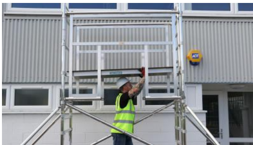
11. Fit 1 trap and 1 plain platform to the 3rd rung down. Making sure the trapdoor is with the ladder section.
