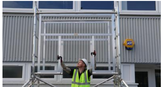
10. Fit 2 Advance Guardrail frames, hooks facing outwards ensuring the top hook is located above the top rung.
