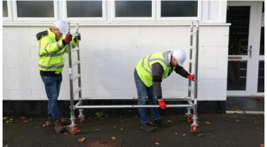
4. Fit 2 horizontal braces to the vertical member of the frames above first rung. Horizontal braces fit on from the inside of the tower facing outwards
