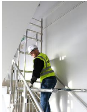
Position the plain portal at the top of your stairs then fit the horizontal braces above the 1st rung.
