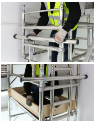
Fit a side prop to the top of each frame, one either end of the tower and then fit your Toe-boards to the tower using the clips.
