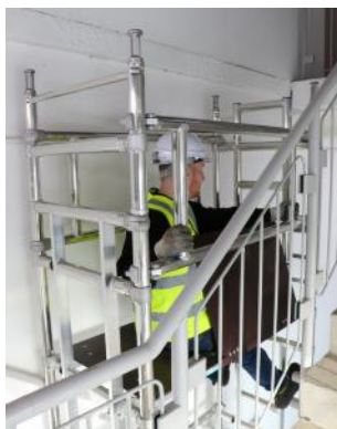
Sitting through the platform, fit 2 guardrail frames, one either side or 4 Horizontal braces 2 either side with hooks facing out. Ensure hooks are fully engaged.
