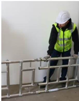
Fit the offset ladder frame* on to the ladder portal frame & position the frame down the stairs.
