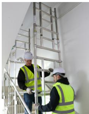
Position the ladder portal at the bottom of your stairs and connect the horizontal braces above the 3rd rung. Level the tower by adjusting the legs.
