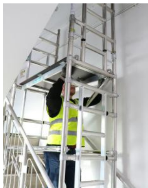
Fit a platform to the 3rd rung of the plain portal frame, trapdoor at the ladder frame side.
