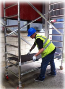
5. Fit temporary* trapdoor platform onto the 2nd rung (if required). NOTE; the 1st permanent platform position is on rung 9, if you can safely reach this from the ground proceed to step 6
