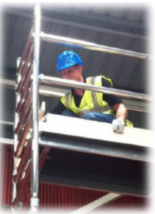
9. Access internally through the trapdoor and sitting on the fixed deck with your feet on the rungs below, fit the mid and top handrails to form a safe guardrail to the vertical tube above the 2nd and 4th rungs.
