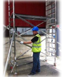
8. Remove temporary platform (if fitted) and fit 2 diagonal braces to the bottom runs running in opposite directions to complete the base.
