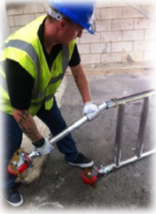
1. Insert Castors and adjustable legs into frames.
