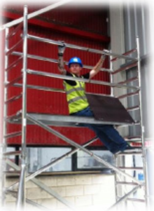
9. Access internally through the trapdoor and sitting on the fixed deck with your feet on the rungs below, fit the mid and top handrails to form a safe guardrail to the vertical tube above the 2nd and 4th rungs.
