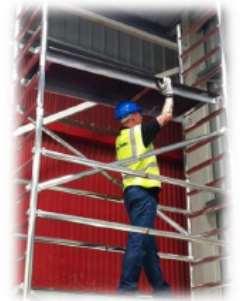
12. Fit next trapdoor platform 1 rung above where the braces end.
