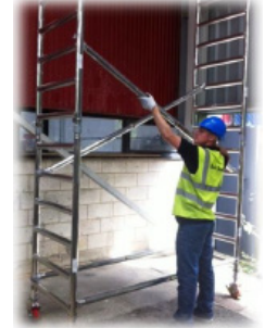
4. Fit 2 diagonal braces to the 5th rungs running in opposite directions to make a cross joining the 2 sets of frames.
