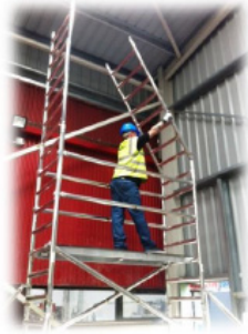
10. Add next set of 8 rung frames and engage the interlock clips.
