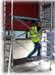
7. Standing on the first platform (if fitted) position the next platform onto the same rung as the diagonal braces.
